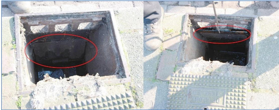
Figure 10 - The baffle plate in gully pot
