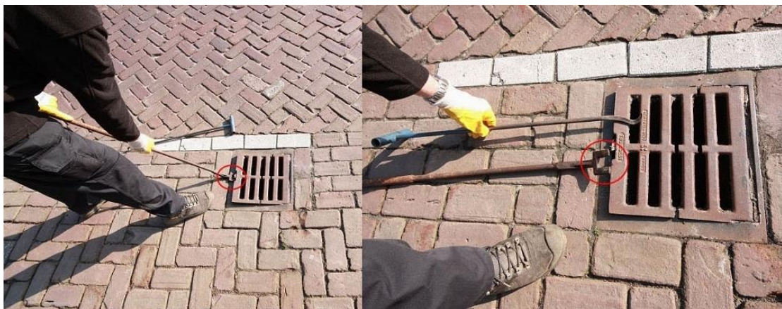
Figure 14 - The other version of the second kind of gully pot in residential area and the special tool
