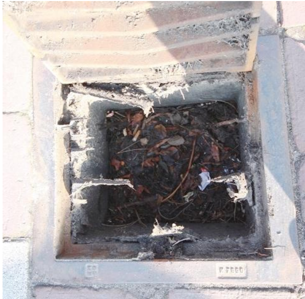
Figure 23 - The gully pot is totally clogged
