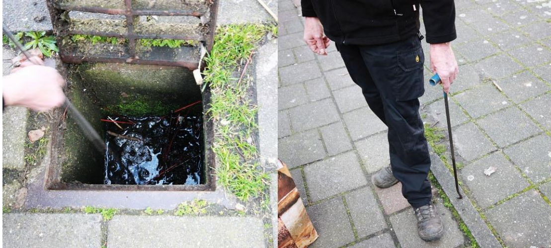
Figure 13 - The second kind of gully pot in residential area and special tool
