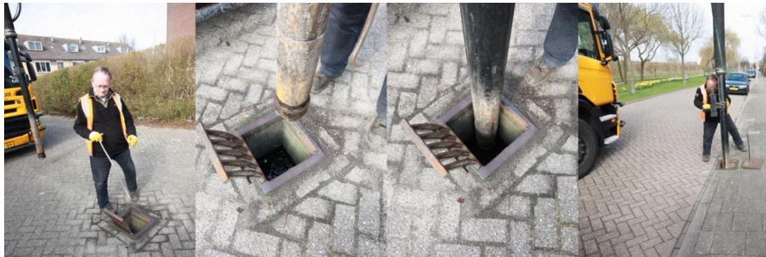
Figure 19 - The suction pipe
