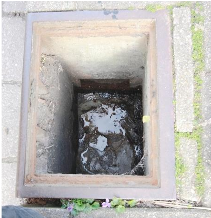
Figure 24 - The concrete stick on the bottom of gully pot
