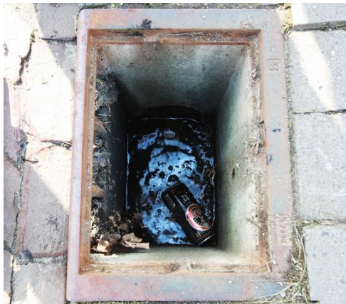
Figure 22 - Beer can in the gully pot
