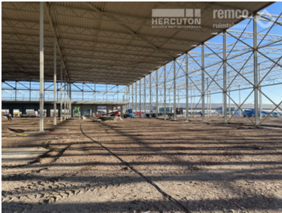
(d) During construction (3)
