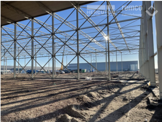
(c) During construction (2)
