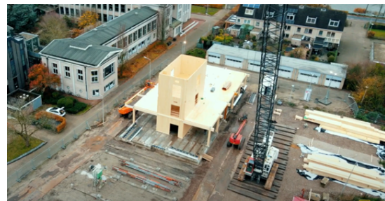
(d) During construction (2)
