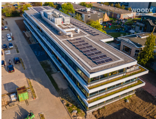
(a) As-built of the building
