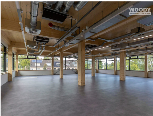
(c) During construction (1)
