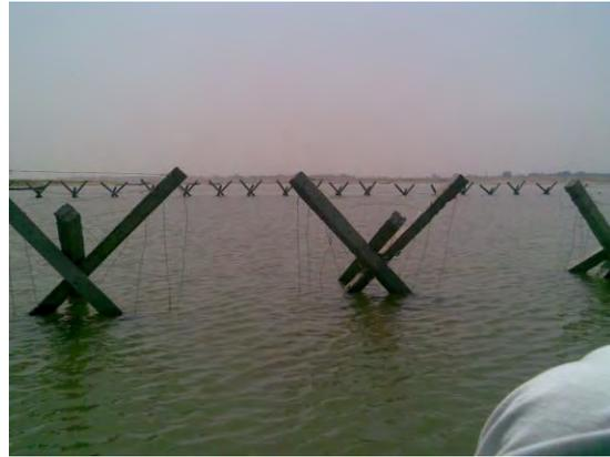
Figure 2.9: Jack Jetty screen for channel closure, from (Nayak et al., 2016).
