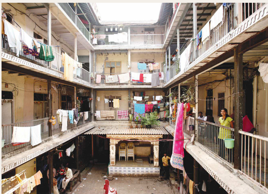
Fig.11 Overlooking balconies and inner courtyards of chawl
