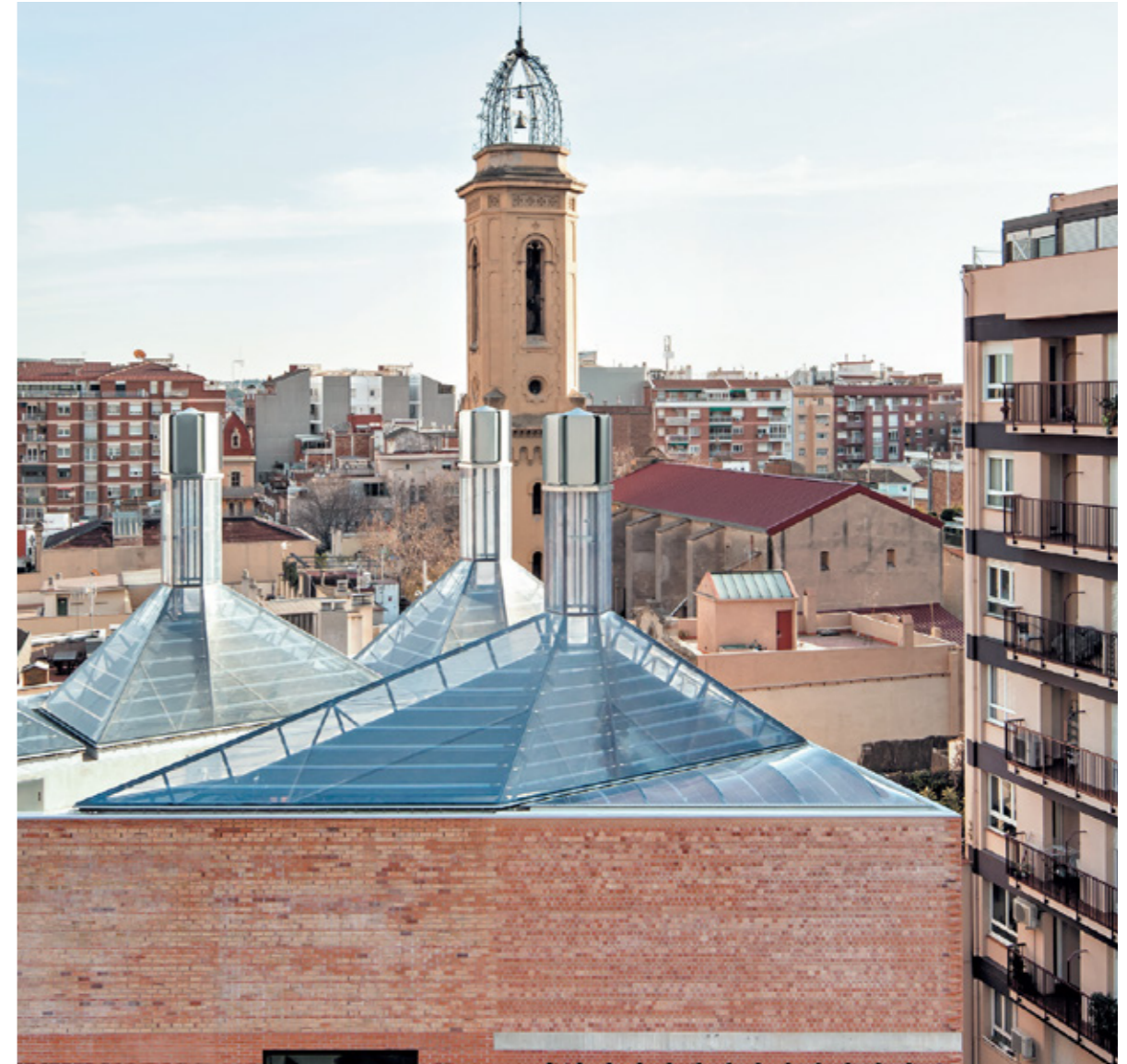
Case: Cristalleries Planell, Barcelona (renovate into civic centre)
