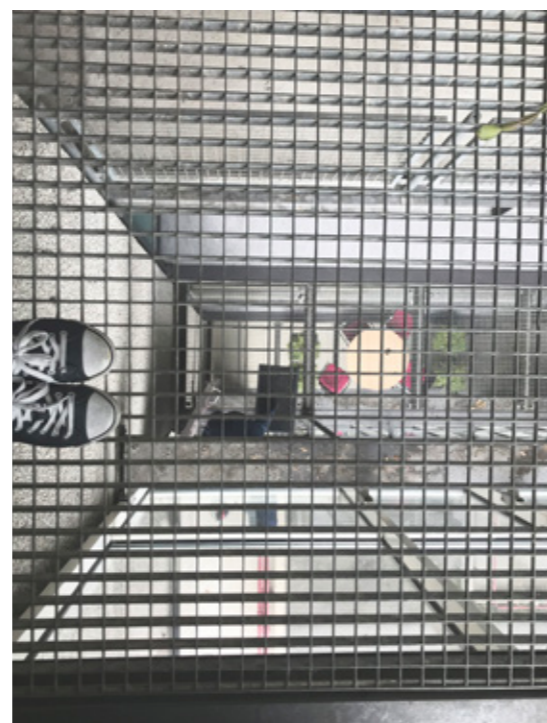
Platform of indoor stairs
