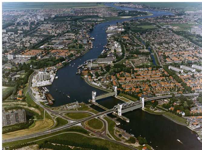
Fig. 2. Hollandse IJssel Barrier. (Image © Rijkswaterstaat, used with permission.)
