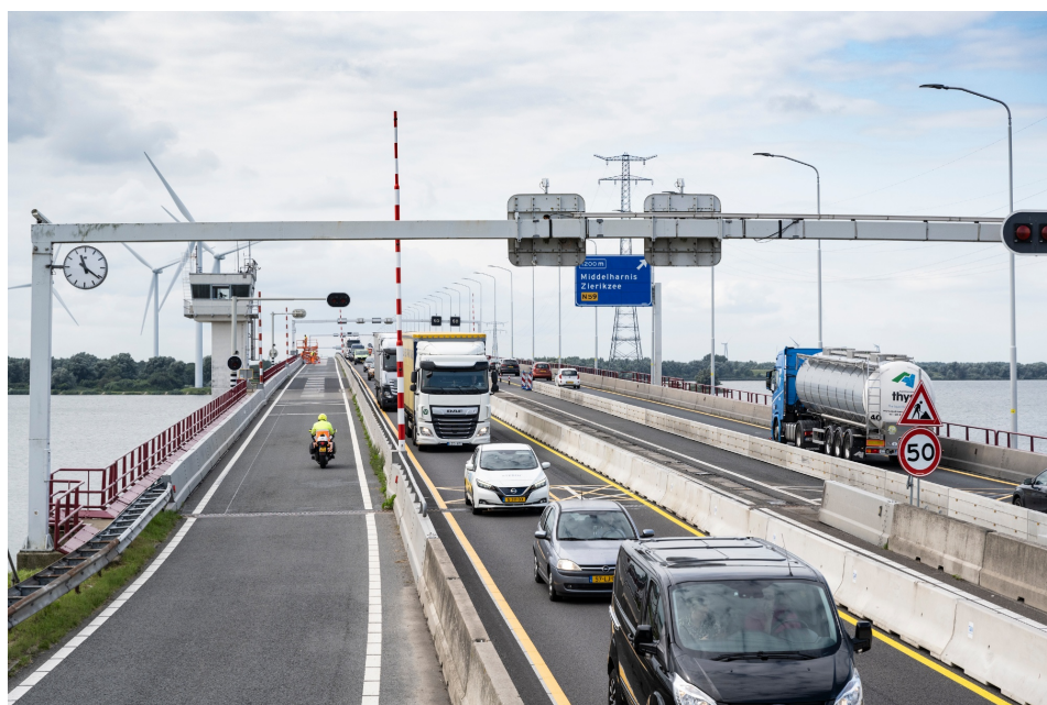
Figure 1.1: A picture of the Haringvlietbrug with the measures taken because of its bad condition (source: Rijkswaterstaat).
