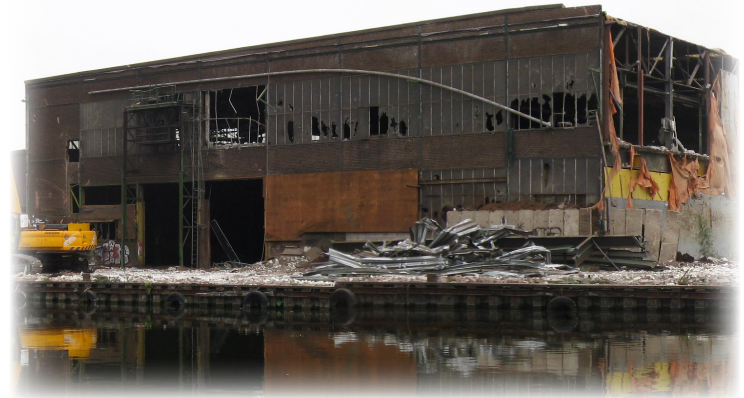
West facade - facing Schie. Demolition summer 2010
