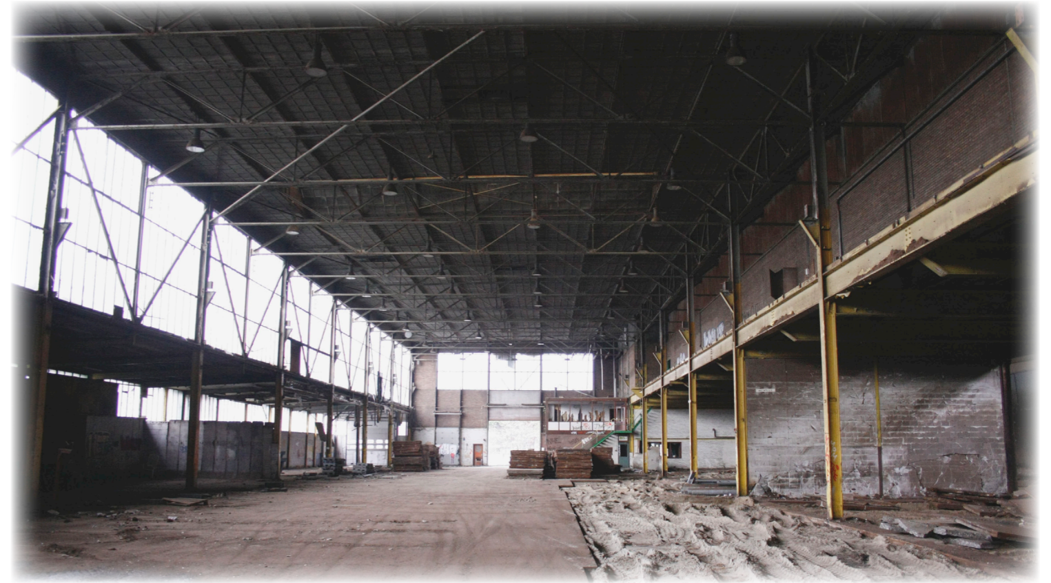
Open part of the hall 20m wide, 110m long.
