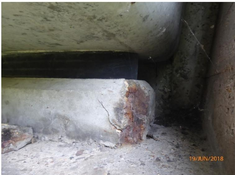
Figure 26 - Wear, mechanical 1
