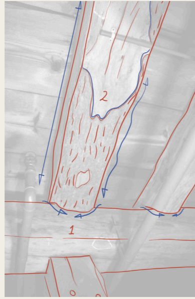
Fig. 3.1.4. Unworked beam in the Munttoren. Photo: Bureau Monumenten & Archeologie, Amsterdam. Analytical overlay: own work.
