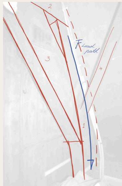
Fig. 3.1.3. Krommer in roof construction, Singel 124. Photo: Bureau Monumenten & Archeologie, Amsterdam. Analytical overlay: own work.
