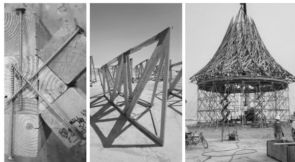
Series of photos from construction site showing - simplicity of the structural elements and different stages of assembly (formatengineers.com, access: 05.01.2022)
