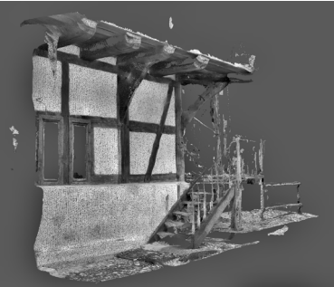
A 3d pointcloud scan of a fragment of an original structure captured on site - the only method of capturing which does not simplify irregularities of the hand-tool system (captured by an author)
