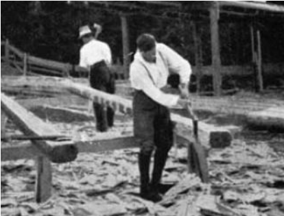
A carpenter using an axe in a process pictured on the infographic above (source: Goodman, 1964)
