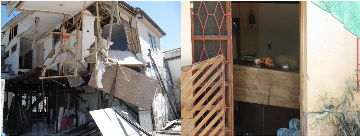
In the city of Coquimbo: homes destroyed.
