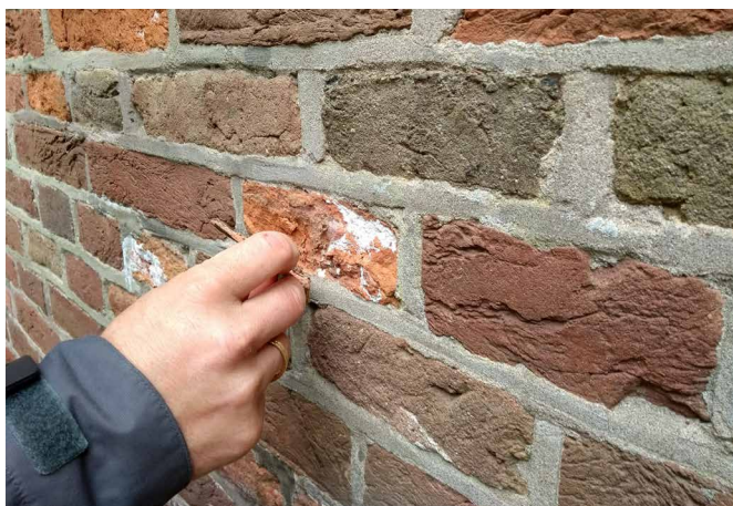
FIGS. 4.14/4.15 Spalling due to salt accumulation beneath the treated layer; the water repellent is still effective several years after the application / Photos: M. van Hunen
