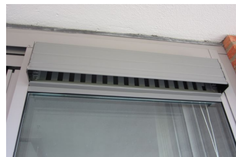
Figure A.39; ventilation grid, from outside
