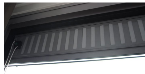
Figure A.38; ventilation grid, from inside
