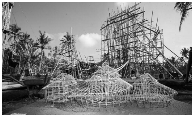
Figure 39-Bamboo scale model as reference for construction.
