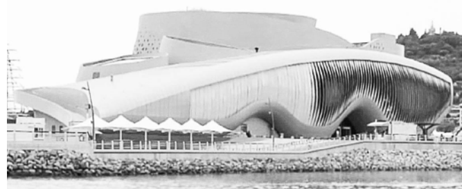
Figure 43-One Ocean Pavillion with open and closed louvers.
