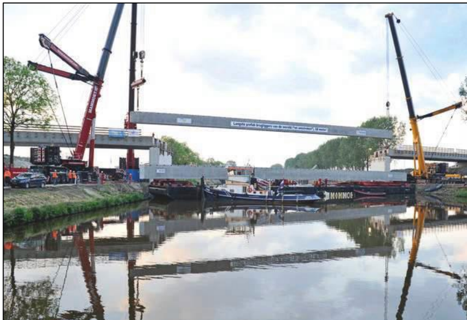
Figure 7.3: Hoisting the 68 meters long prefab beam into final position [23].
