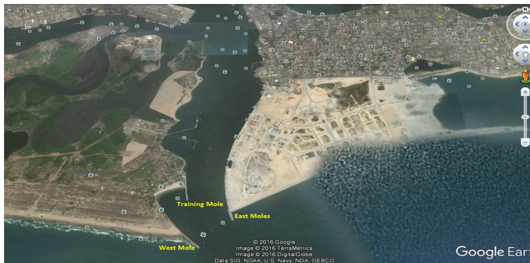
Figure 2.2. Modified Google earth image showing Tidal inlet on Lagos coast Nigeria. Figure above shows the coastline by 2006, figure below shows the coastal modifications made behind the East mole (Atlantic City that extends the bar beach coastline seawards).
