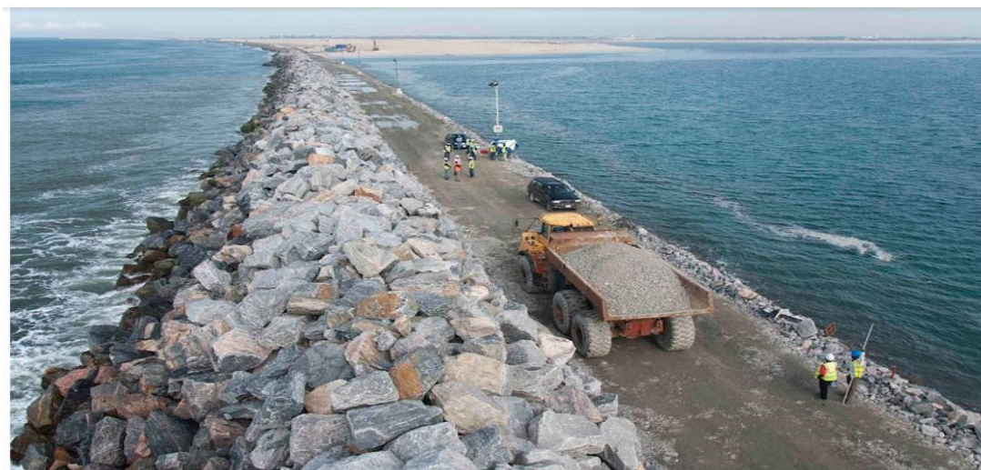
Figure 2.3. Eko Atlantic City barrier wall to protect against erosion from waves. It is made of stones piled 15 meters (42ft) high and topped with concrete accropodes. Retrieved from: http://www.ekoatlantic.com/latestnews/press-releases/a-city-rising-from-the-sea-the-dazzling-eko-atlantic-project-in-nigeria/
