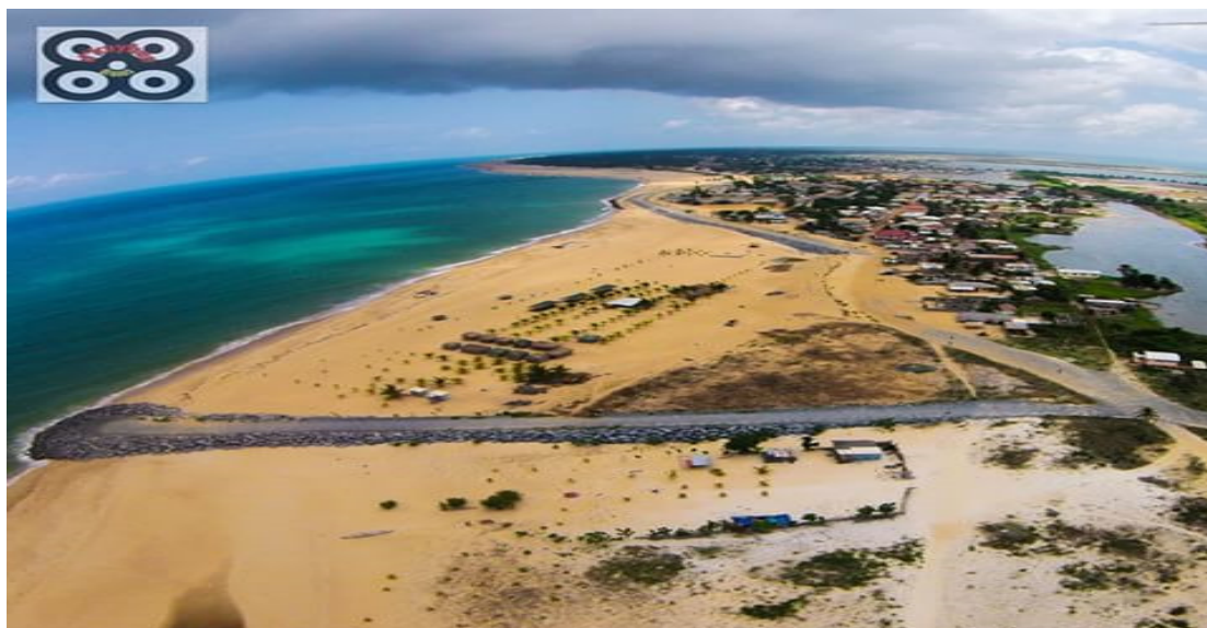
Figure 2.5. Groin constructed as part of the Keta Sea Defence system on the East coast of Ghana. Retrieved from http://www.imgrum.net/media/978781727019795732_37222592
