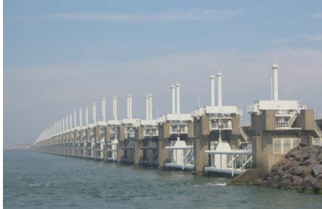
Figure 1.1 Eastern Scheldt Storm Surge Barrier (Šiman, 2008)
