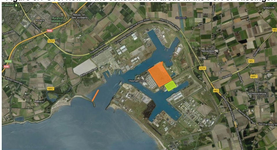
Figure 6.1 Overview of the construction areas in the Port of Vlissingen
