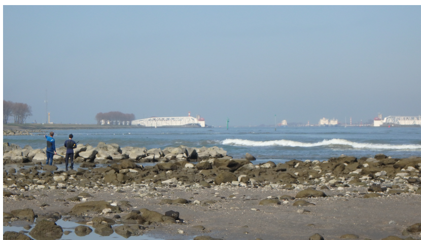
Figure 4.3: Ship waves breaking in the adjacent groyne.
