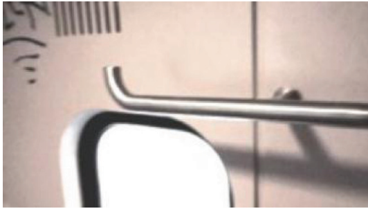
Fig. 15. Hook 2: actually, mentioned for another purpose, positioned at the height of 1,700 mm from the floor.
