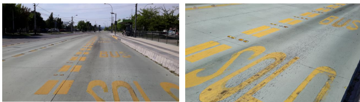
Fig. 7.3.9. Bus corridor “Avenue Vicuña Mackena” after 9 years in-service
