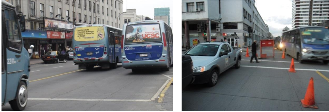
Fig. 7.4.2. JPCP with short slabs at a bus lane in Concepción city, Chile (Pradena and Houben, 2014a)
