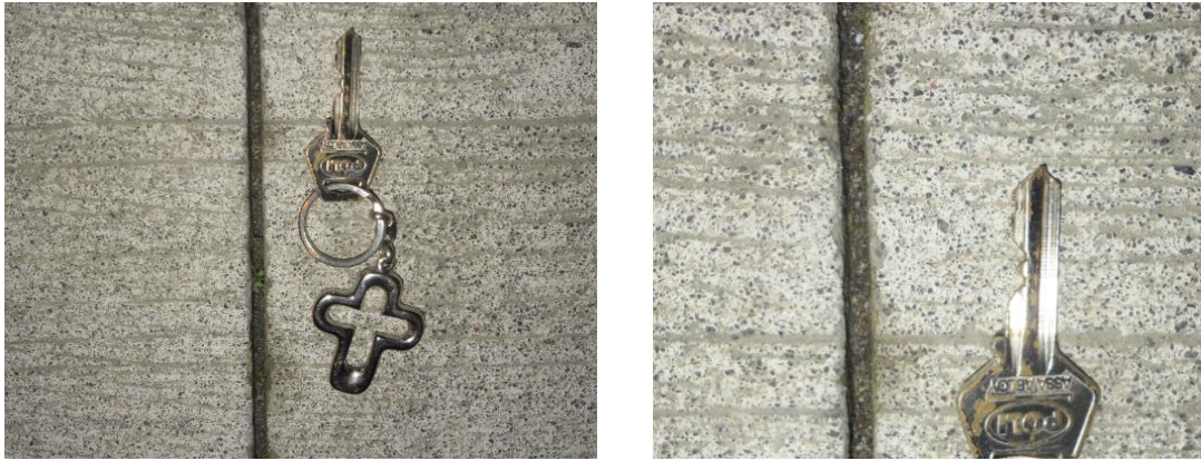
Fig. 7.3.6. UnJs filled with fine incompressible material (saw-cut 4 mm) (Pradena & Houben, 2015a)
