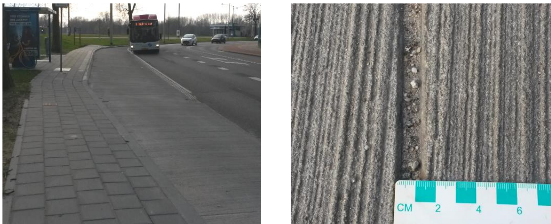
Fig. 7.3.2. Sealed joints contaminated with incompressible material at bus stop, Arnhem city, the Netherlands.
