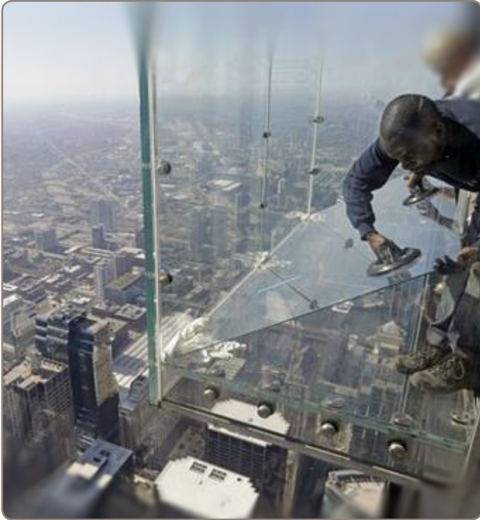
Figure 15: Replacement of sacrificial layer
