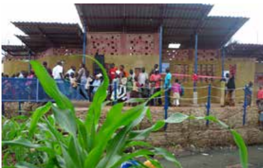
Multipurpose building (KDI, 2018)
