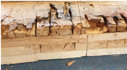
Deterioration causes loss in mass and stiffness
