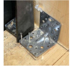
Nail withdrawal at angle brackets
