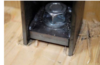
Wood crushing under hold-downs
