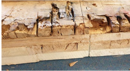
Deterioration causes loss in mass and stiffness
