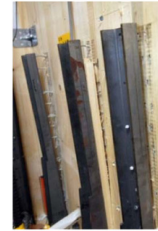
Nail failures at hold-downs
