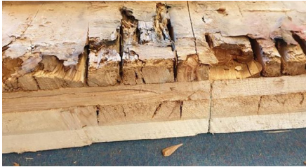
Deterioration causes loss in mass and stiffness
