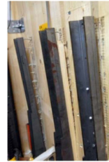
Nail failures at hold-downs
