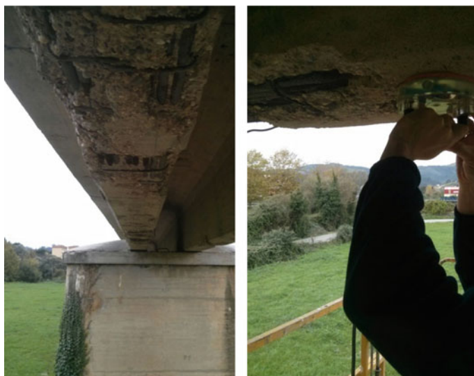
Fig. 2 Selected areas during the repair phase
