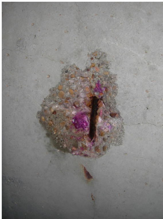
Fig. 6 Picture of the corrosion rebars in the structure A in a carbonation zone
