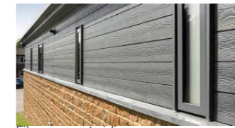
Fiber cement siding
