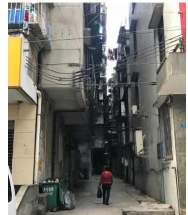
Figure 71: 80s and 90s old residential buildings
