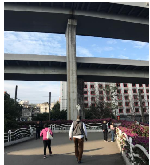
Figure 74: People can only use a few overpasses to cross traffic barriers.
