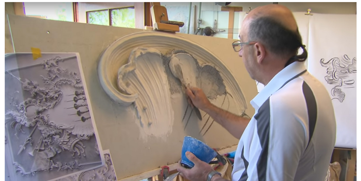
Figure 15 Salvater applying the rough shape of the missing part of a damaged ornament with a trowel. Notice the photographs and sketches he is using as reference. Adopted from https://www.youtube.com/watch?v=8_dwEbF-Nil
