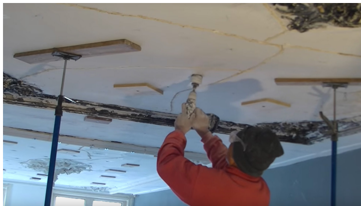
Figure 182 Temporary supports underneath a stucco ceiling. Adopted from: https://www.ornamenten-restauratie.nl/ornamenten-plafond-vastzetten/
