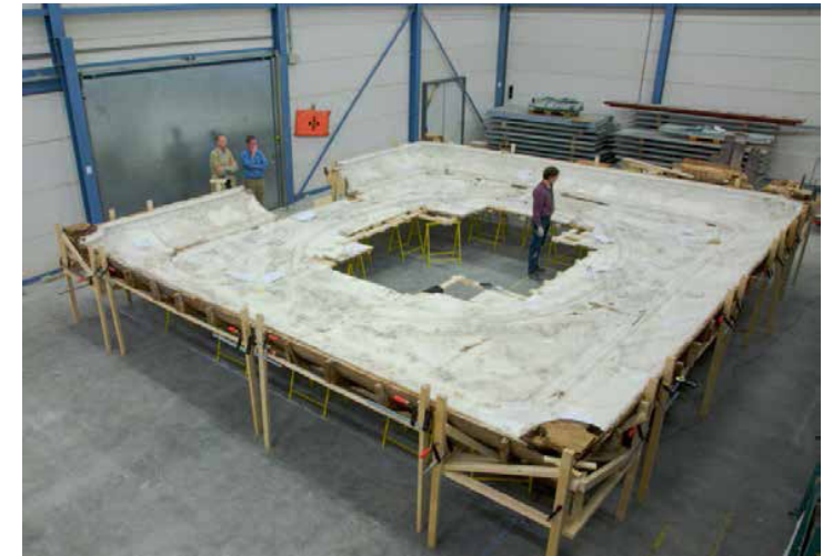
Figure 14 Cut out ceiling of the Beuningkamer brought to a workshop. Source: R. Klein Gotink.
