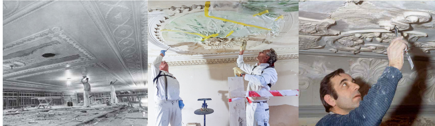
Figure 16 On-site stucco ornament restoration work. Sources: tbaibouw.nl, (Geerken & Freling, 2010)
