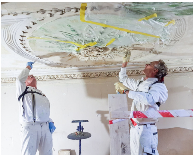
Figure 10 Restoration of stucco ornament in Huize Nolet. Source: https://www.tbafbouw.nl/
