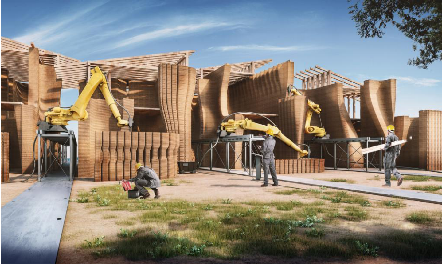
Figure 209 Rendering of digitally fabricated earth & timber housing by IAAC. Adopted from: https://iaac.net/educational-programmes/applied-research-programmes/otf-3d-printing-architecture/
