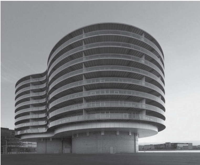
Frøsilos in Copenhagen (Nielsen, 2010)
