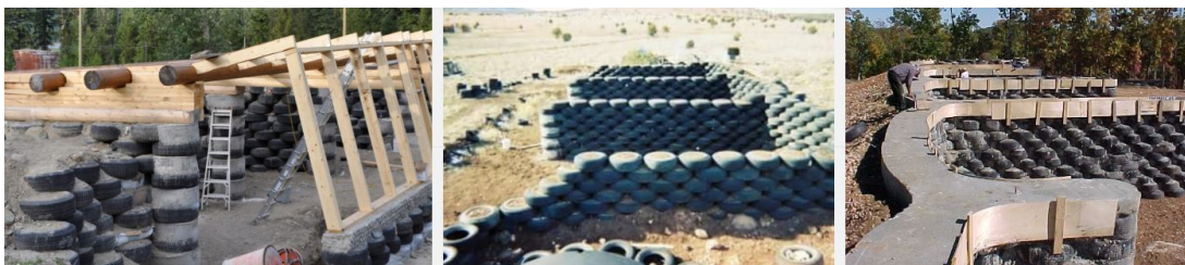
Figure 14.4: Examples of tire walls in Earthship buildings
