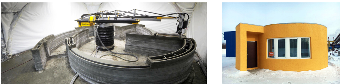
Figure 2.19: Printed house by Apis Cor (Sakin and Kiroglu 2017)
