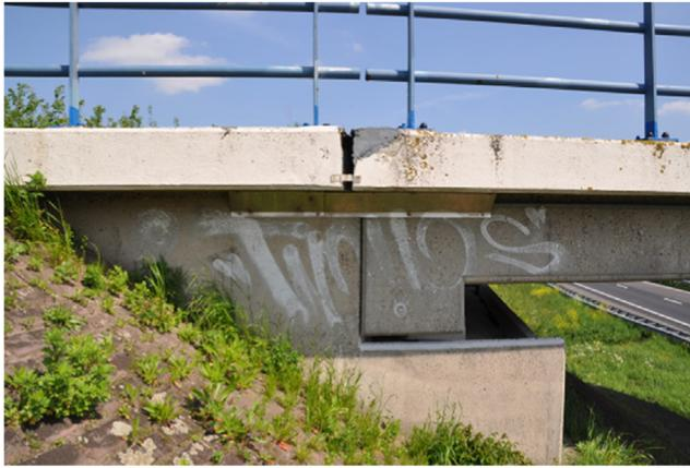
**Figure 6.7** Closing of the expansion joint between the slab and the abutment.
