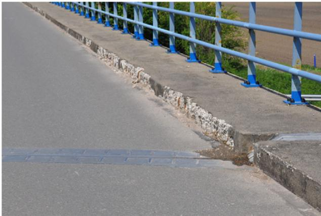
**Figure 6.6** Concrete deterioration of the sidewalk.
