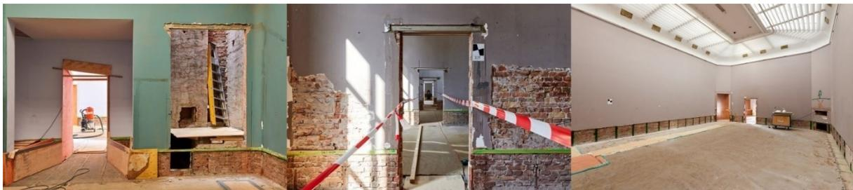
Figure 3-1: Current state of the Van der Steurgebouw after removal of asbestos (photographs by Aad Hoogendoorn<sup>5</sup>)
