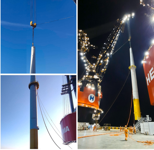
Fig. 3. Tugger lines attached to the OWT tower during installation: Active tugger line attached on the hook block (top left), passive manual tugger line attached on the skybox location on the lower tower (lower left), and overview picture (right). Sensor locations are detailed in Fig. 2.
