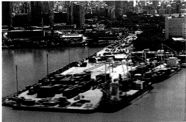
Figure 1-6 View of TRP, pier 1
