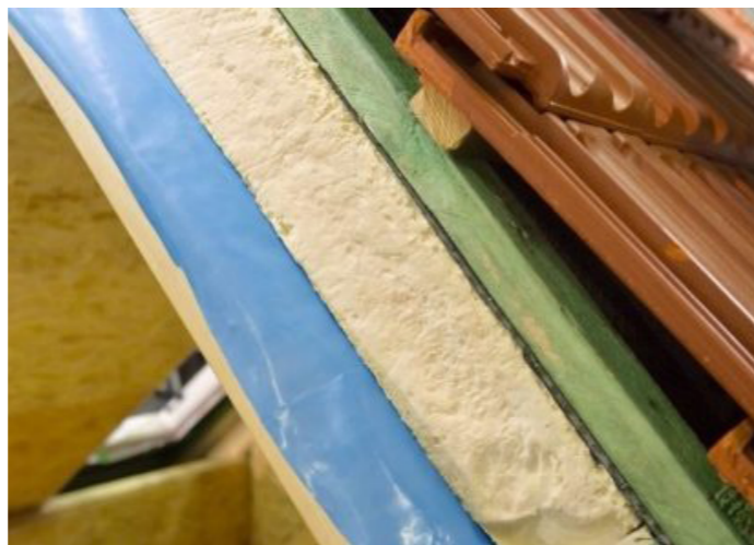
Figure 16 Layers of insulation for a pitched roof.
