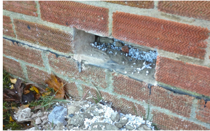
Figure 11 Inspection for debris in the cavity.
