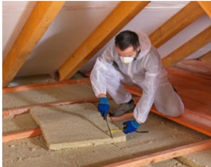
Figure 15 Insulation between the wooden beams.
