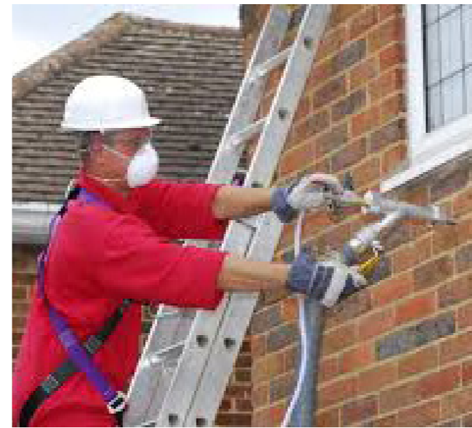
Figure 10 Cavity insulation in the cavity through a hole.
