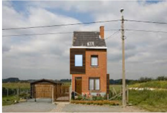
Figure 7 Project's front facade. (cityzen-smartcity.eu)
