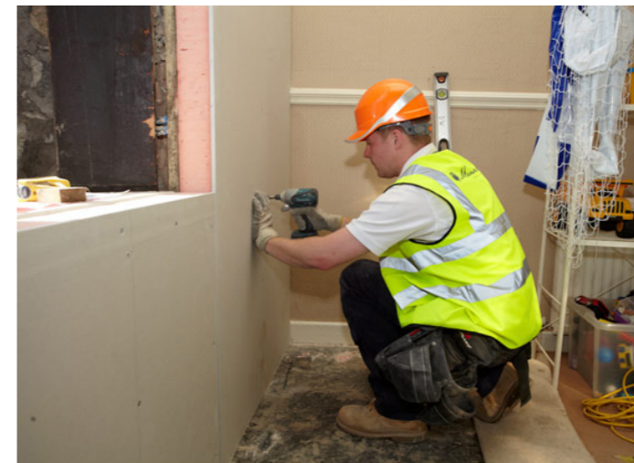
Figure 14 Internal wall insulation application.
