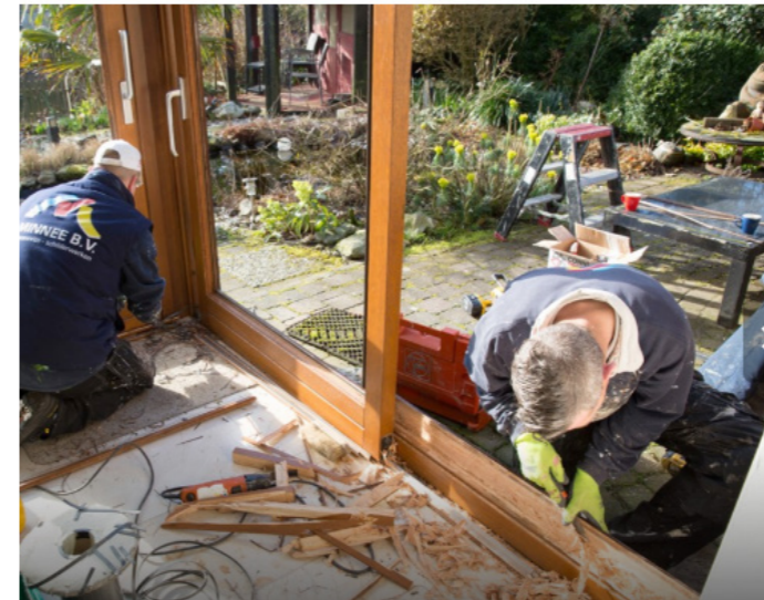
Figure 17 Preparing the frames for the thicker glass.
