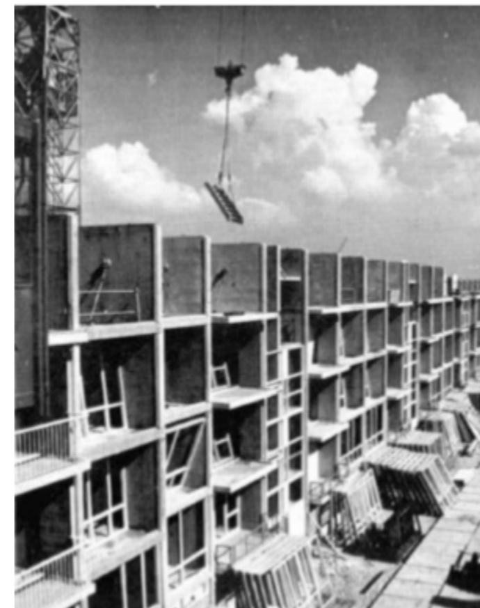
Fig 1 Example of the system construction, (Bouw hulpgroep, 2013).
