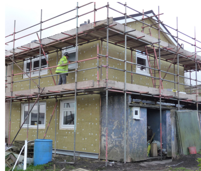
Figure 13 External Wall insulation application.
