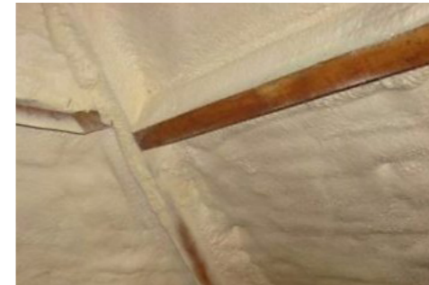
Figure 20 PUR inside the pitched roof.
