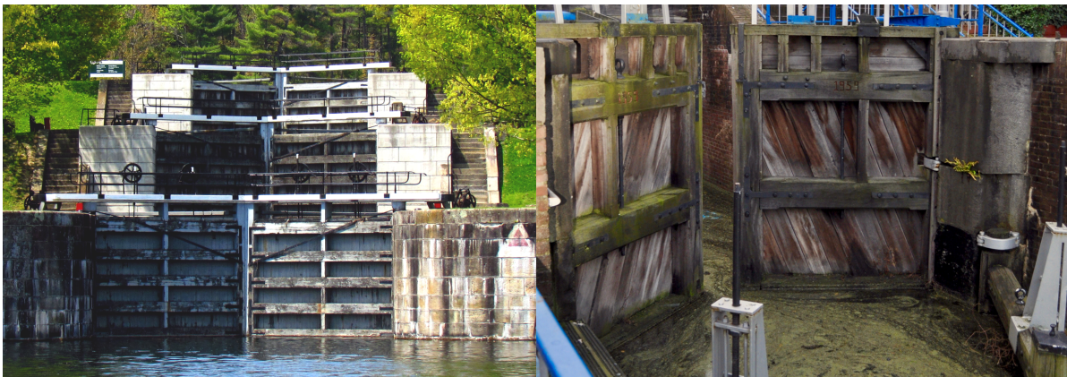
Figure 1.1: Mitre gate in use, "Jones Falls Locks" [1] (left) and "Monstersche Sluis" (right) with the drawn the top and side views.
