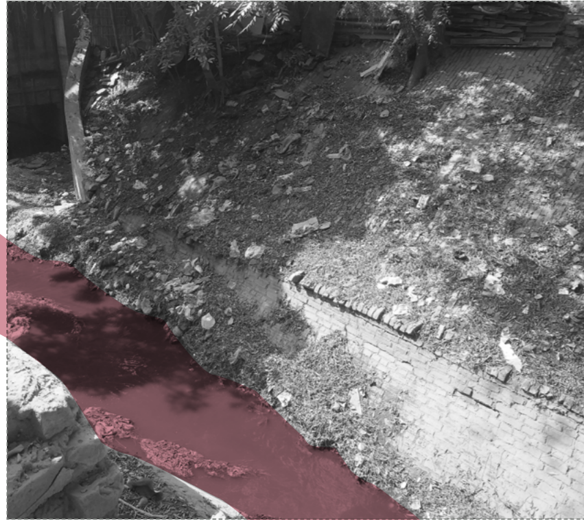
1. Lack of Infrastructure (Sewage and Water Supply)
