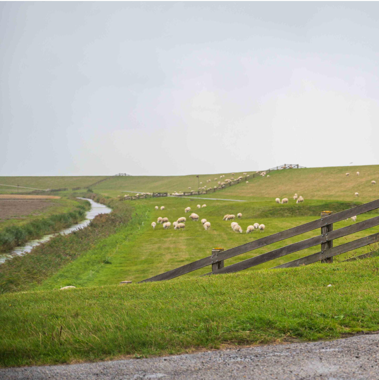
Friesland Sea Dike, 2022. Photo: Xinjian Jiang.
