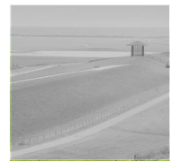
Old Sea Dike
