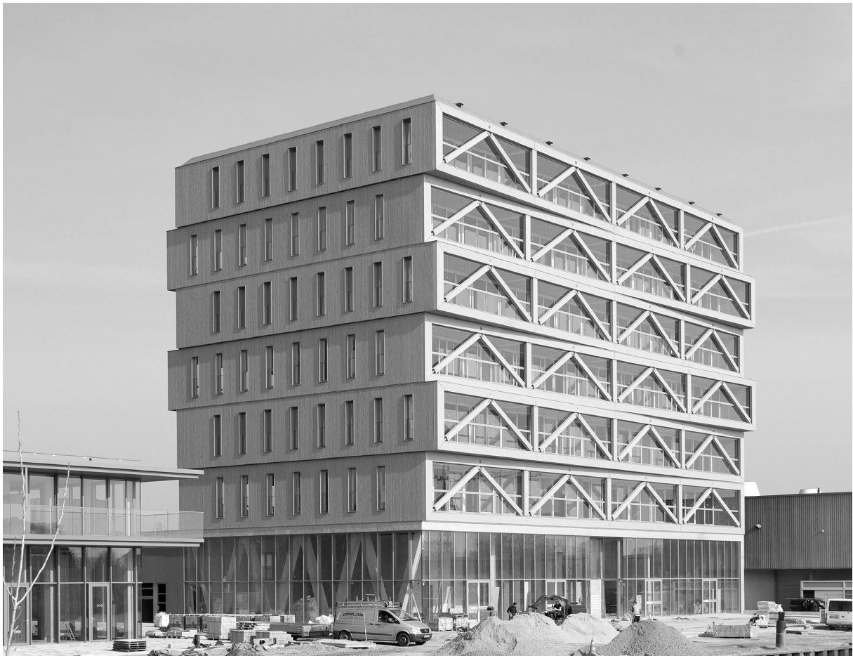
14 Photograph 3: Patch-22 SouthWestview (v.d. Burg, 2016)
