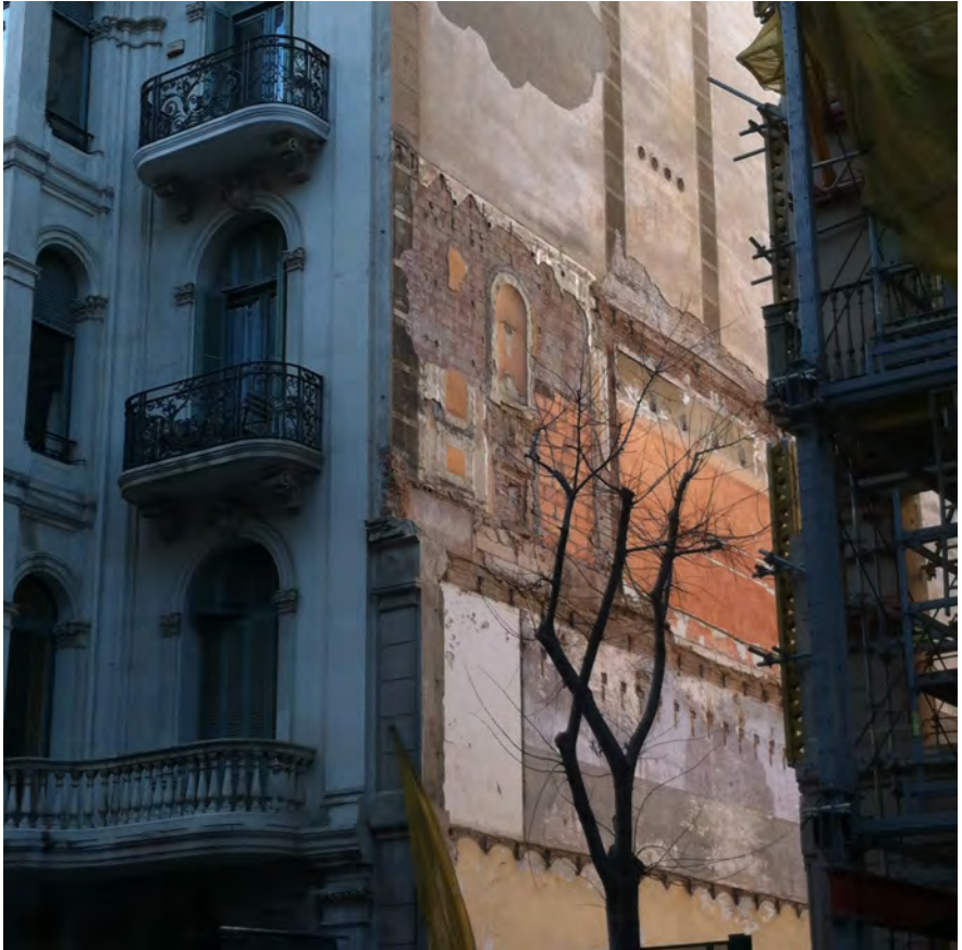
fig. 1 empty plot in Barcelona, 2014 Due to the demolition of a dwelling building, a void emerges in the street facade, allowing light to flow in from another angle and revealing previous layers of use.
