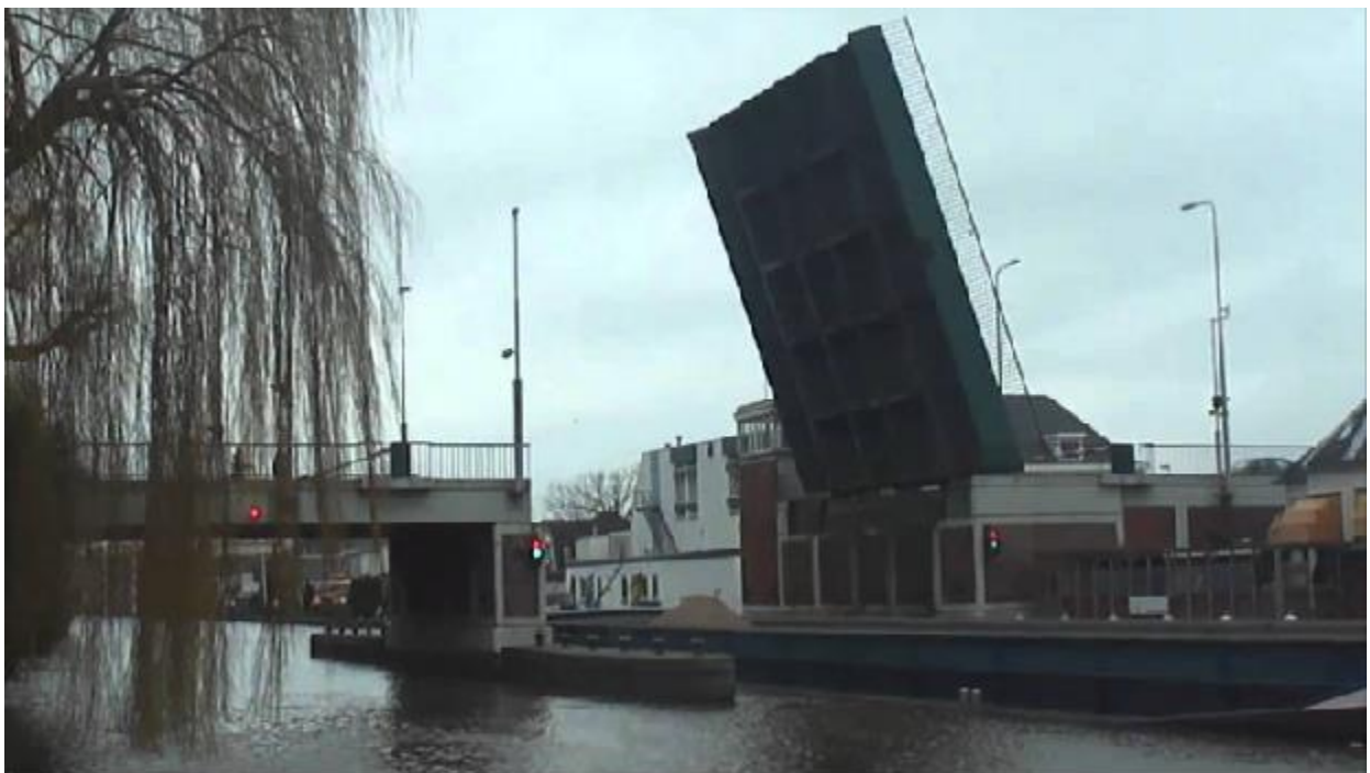
Figure 4: View of the Koningin Julianabrug in open position 10
