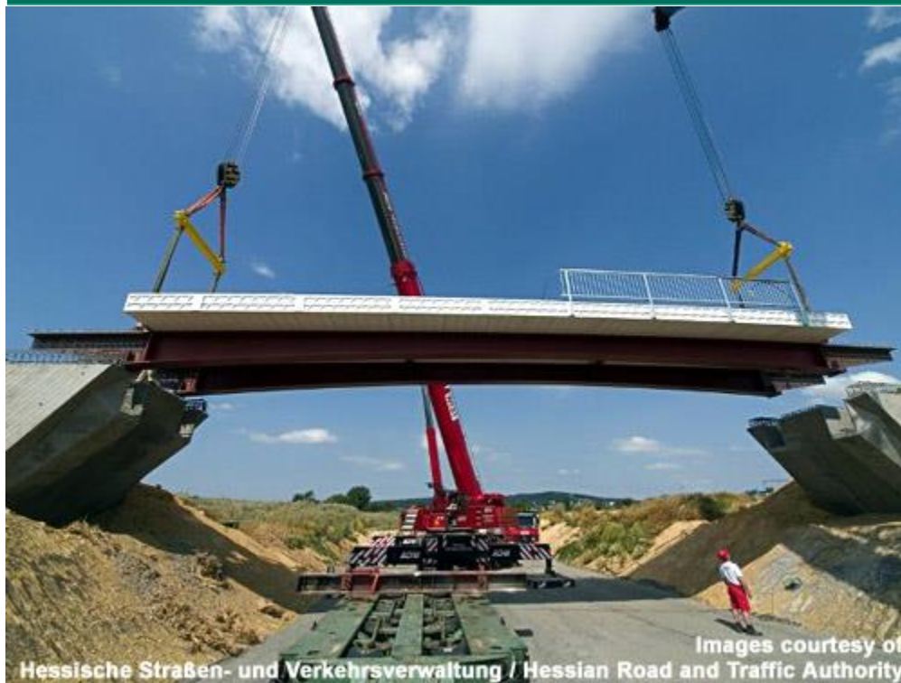
Figure 92: Installation of Friedberg Bridge 131
