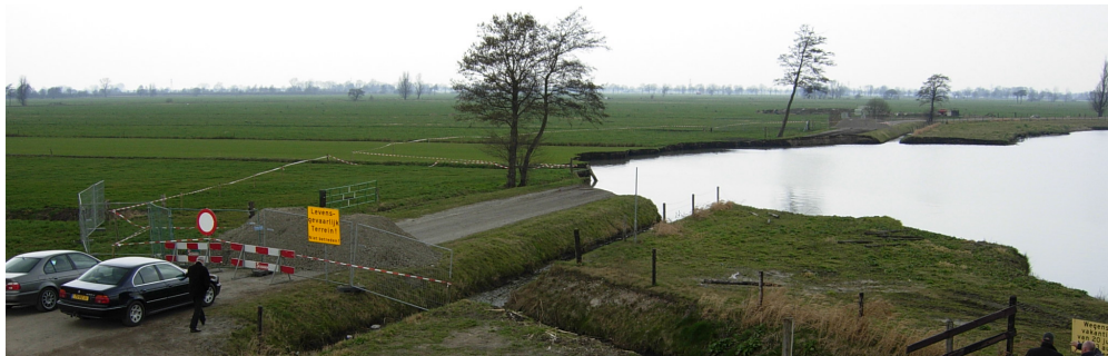
Figure 1. A lake border damaged by the unstable breaching process at Hooijdijk, 2008. (Source: D.R. Mastbergen)
