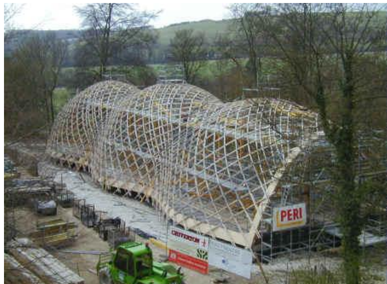
Figure 2-26: Construction of Gridshell (Source: Buro Happold)
