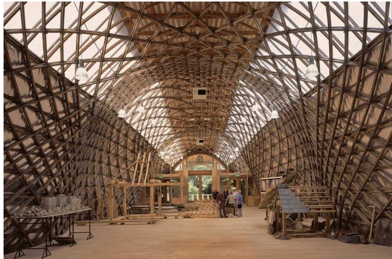
Figure 2-25: Downland Gridshell Interior (Source: Buro Happold)
