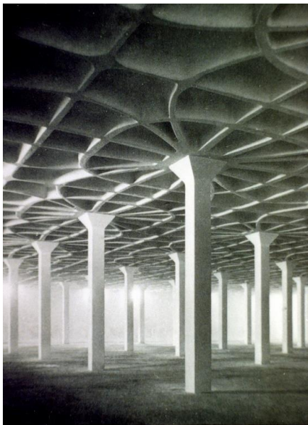
Figure 2-2: Gatti Wool Factory Roof (Winslow, 2010)
