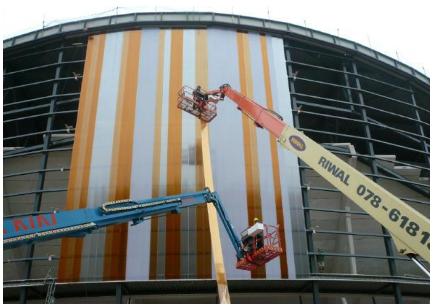
Omnisport in Apeldoorn with polycarbonate facade panels 23 m height ( http://rodeca.nl/ )
