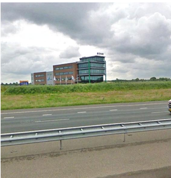
View of the office building heading south on A28
