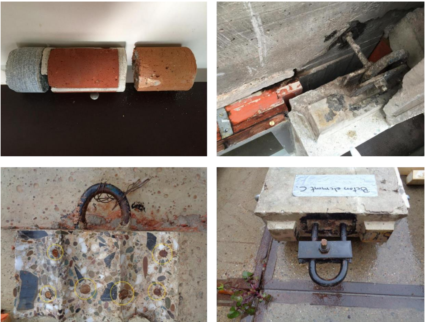
Figure 30 - Facade elements and connections, (Peutz DGMR, 2015)
