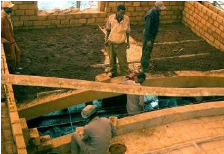
FIGURE 07: Catalan vault floor slab at SUDU project, Ethiopia, with lightweight stiffening walls and compacted fill. Image retrieved from López López, D., Van Mele, T., & Block, P. (2016). Tile vaulting in the 21st century. Informes de La Construcción , 68(544), 162. https://doi.org/10.3989/ic.15.169.m15
