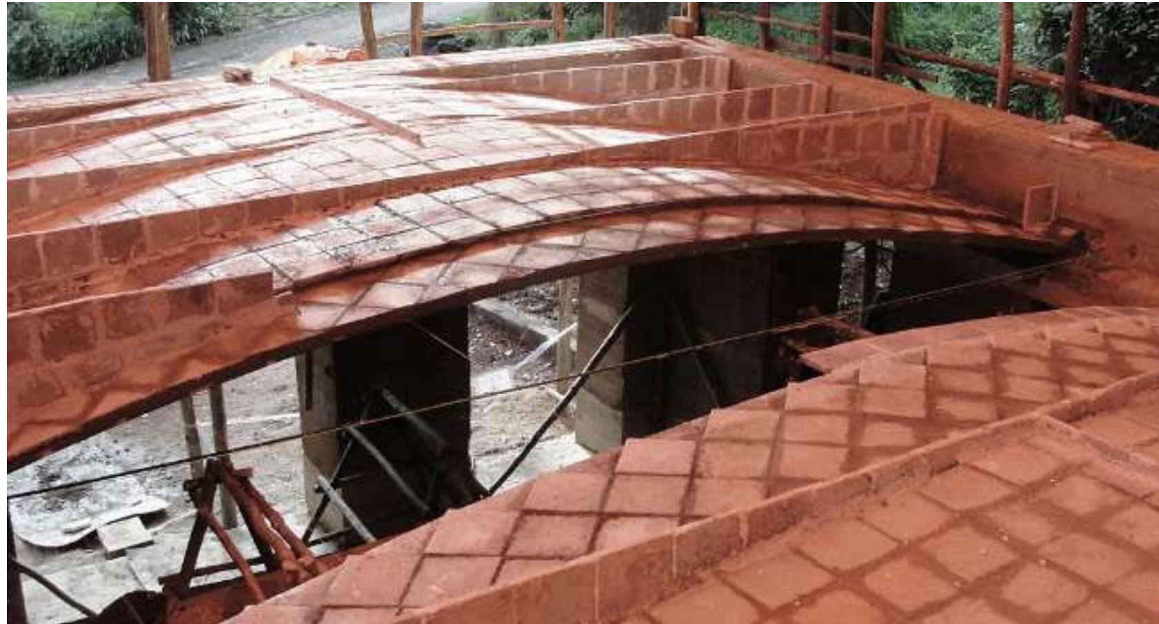
FIGURE 04: Catalan vault floor slab at SUDU project, Ethiopia with lightweight stiffening walls. Image retrieved from López López, D., Van Mele, T., & Block, P. (2016). Tile vaulting in the 21st century. Informes de La Construcción , 68(544), 162. https://doi.org/10.3989/ic.15.169.m15
