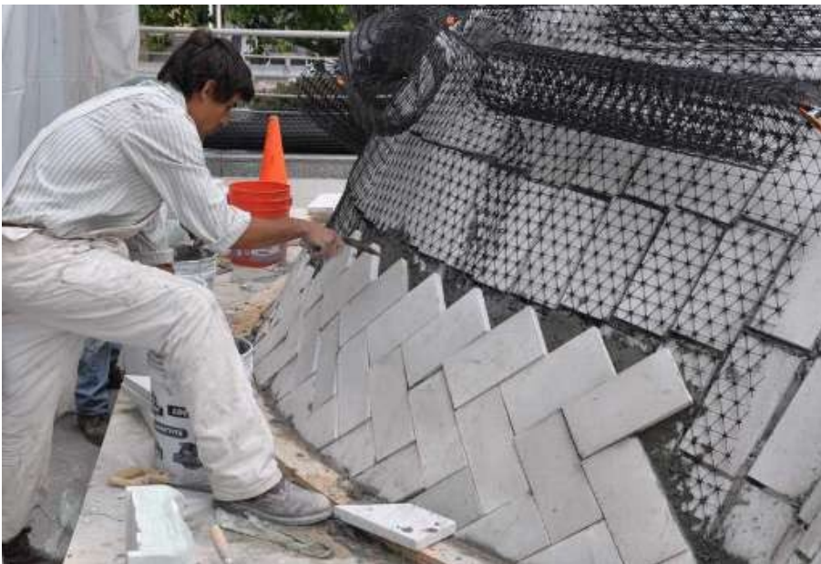
FIGURE 05: Geogrid embedded in between mortar layers and tiles, for reinforcement against seismic loads, in the Bows Centre, Yerba Buena Centre for the Arts, in San Francisco, USA. Image retrieved from Ramage, M. H., & Dejong, M. J. (n.d.). Design and Construction of Geogrid-reinforced Thin-shell Masonry.
