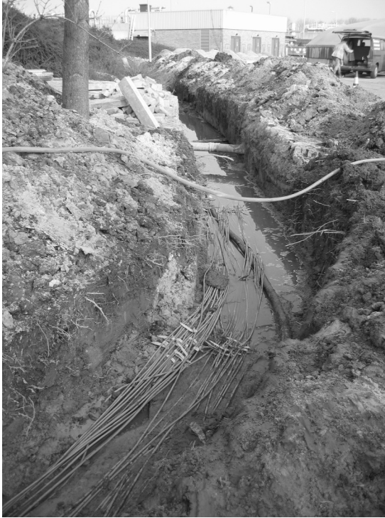
Figure 5.1: The trench with dozens of cables.
