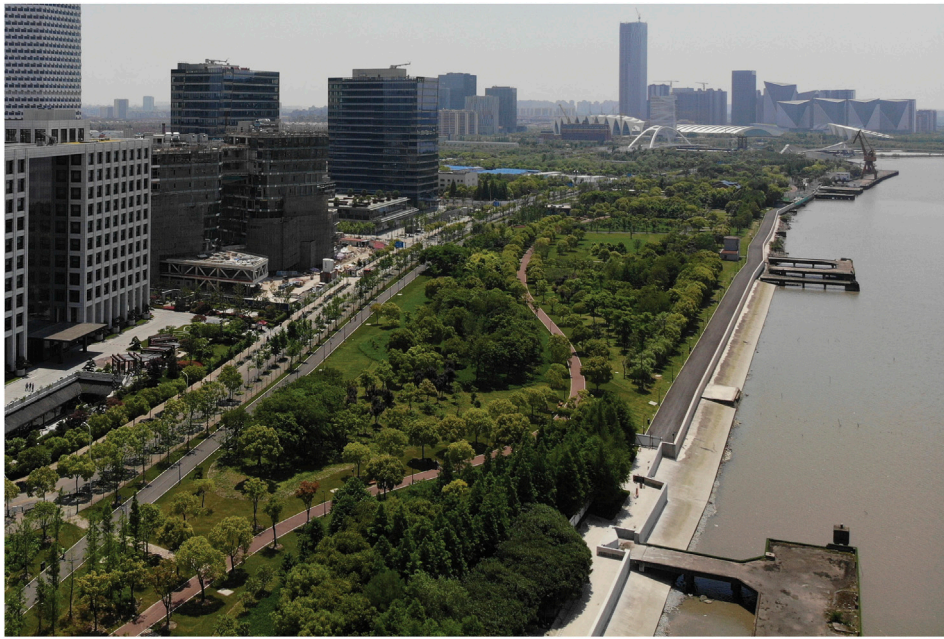
FIGURE 3 | Hard embankments in new ecological park along the Huangpu River (Photo by author, September 2020).
