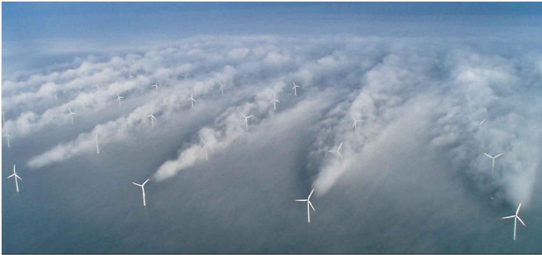
**Figure 1-1:** The Horns Rev offshore wind farm near Denmark under foggy weather conditions. The flow wakes formed by turbines extracting energy from the wind are clearly visible. [10]
